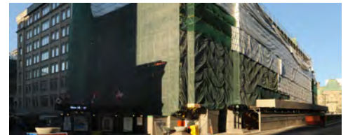
144 Wellington Street, Ottawa, during construction.
